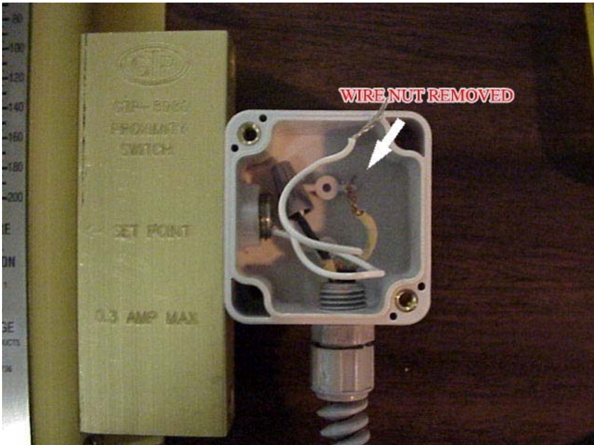
Remove one of the two wire nuts. It does not matter which one.
