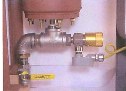
Note: The IS relay may be wired by the installer to the deadman system to stop fuel flow, provide an audible warning, and/or provide a visual signal such as a red light labeled “water in sump.”
